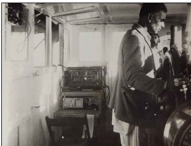
An inside view of M. V. Mahindra (1963) where a crew member is seen at the steering control. On the left is the console for navigation, with the Decca receiver on top and the audio equipment below. (Photo courtesy: Mr. V. C. Mohan)
