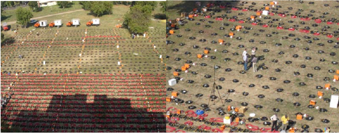
Spread on the Ground during installation & commissioning
