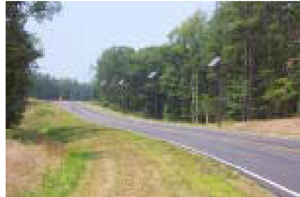
Figure 4. Photovoltaic Domestic and Streetlights.
