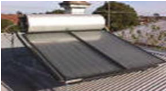
Fig. 1 Solar Flat Plate Collector
