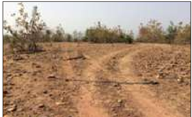
Fig. 10: Safe Guarding line cable with road mats
