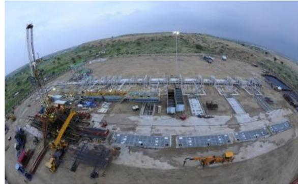
Figure: Completed Mangala Wellpad with Wells in Cellar
